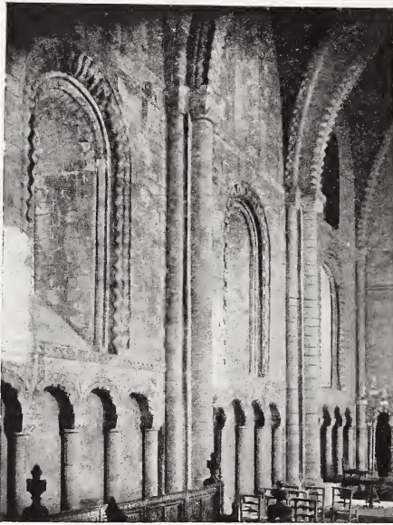
114. STOW, LINCS. ARCADE IN CHANCEL
